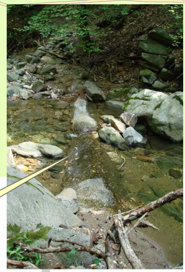
Pipe Encasement visible at Stream Bed
